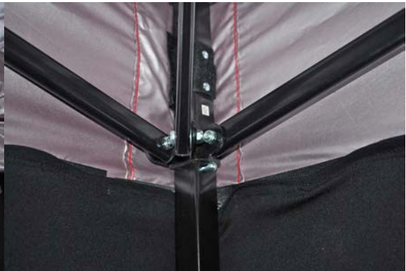
Figure 6: Tent frame needs to be above this button
